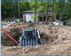
An off grid rural property owner installed 2 x 6500L Carat tanks outfitted with Optimax self-cleaning filter package and a Grundfos SBA-45 pump. The system will collect rainwater from the 900 sq. ft. roof of a new garage building. The water will be used to water landscaping and to supply a wash station in the garage. With 2 tanks the owner installed the filter package in one tank and the pump in the other tank to ensure ease of access for any future pump maintenance.
